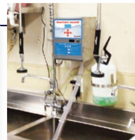
Unit mounted above sink with solution discharge tube placed in sink.
